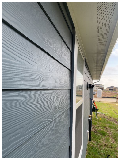
TRIM APPLICATION FOR WINDOWS, DOORS & OTHER OPENINGS Flashing over trim is required per code for all installation methods. (Figure 14)
